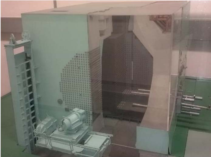
Figure 4.4: Scale model of BR1 with visible graphite pile.
