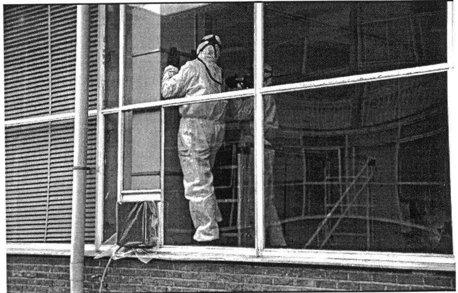
Photo 2 : Dismantling of ventilation pipes
