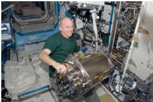
Figure 5: NASA astronaut Jeffrey Williams installs the Urine Processor Assembly/Distillation Assembly in the Water Recovery System rack on the ISS (Credit: NASA)
